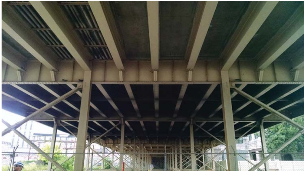
View under the Bridge from the 11 th Street looking West
