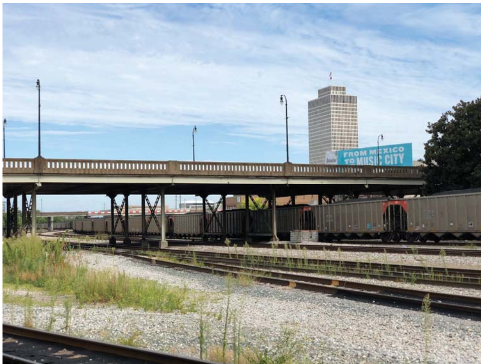
View of Bridge over CSX Rails from South
