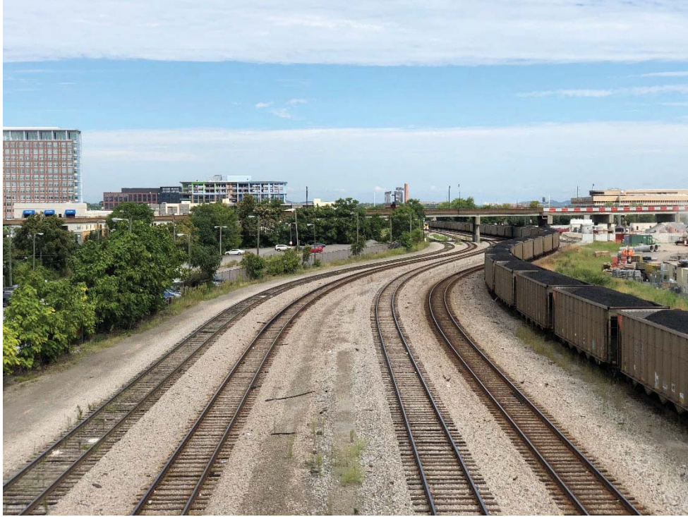
View to North over CSX Rail
