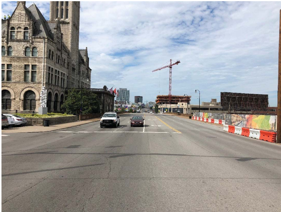
View of Bridge from East Approach
