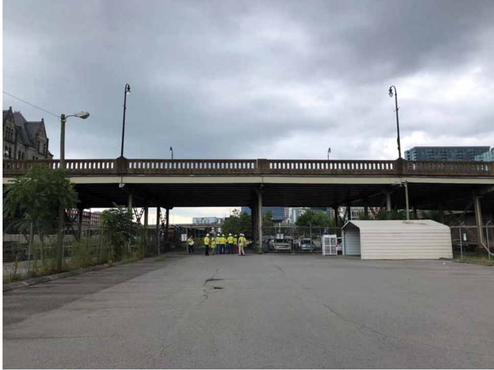
View of Bridge from North
